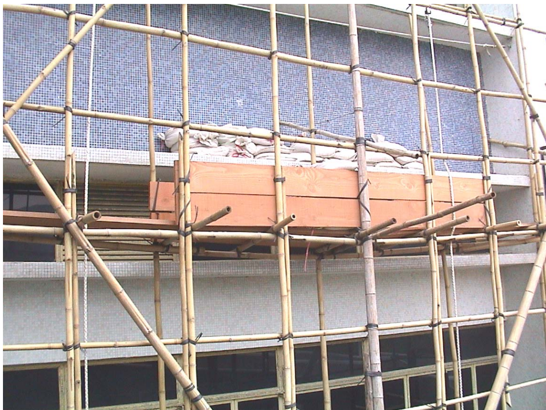
Figure 1.3 Typical configuration of a double layered bamboo scaffold
