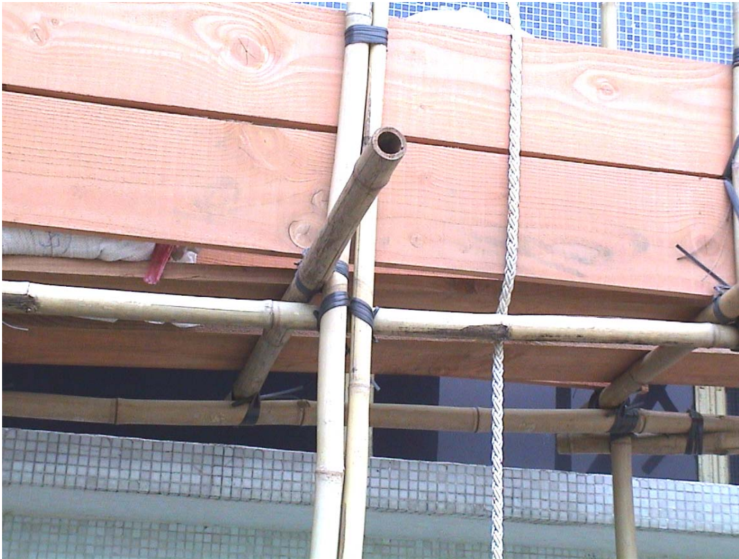
Figure 1.4 A close-up on the ledger-post connection
